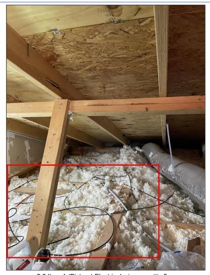
2.8 Item 1 (Picture) Electrical wires on attic floor
